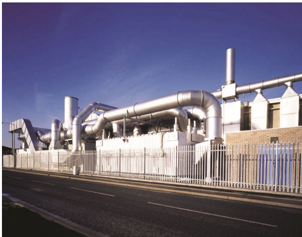
Caption: Transcontinental Advanced Coatings is extending ABB's digital condition monitoring solution to an entire production line following a successful pilot study on a critical oxidizer (pictured)
